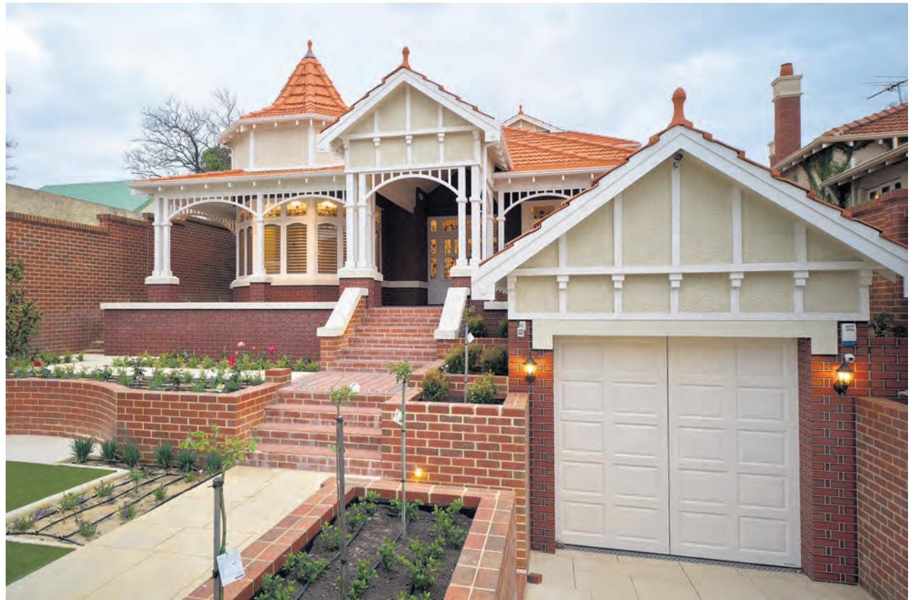
Many traditional features such as tuckpointing, texture render and feature gables reference the Federation style.
